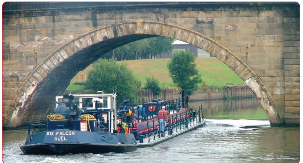
Beauforth House is situated close to the area from which Ferrybridge takes its name
