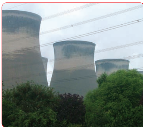
Nearby Ferrybridge power station is one of the biggest producers of electricity in Yorkshire and Humber
