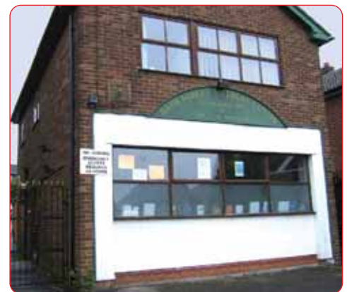
Bath Street Practice in the West Midlands town of Sedgley
